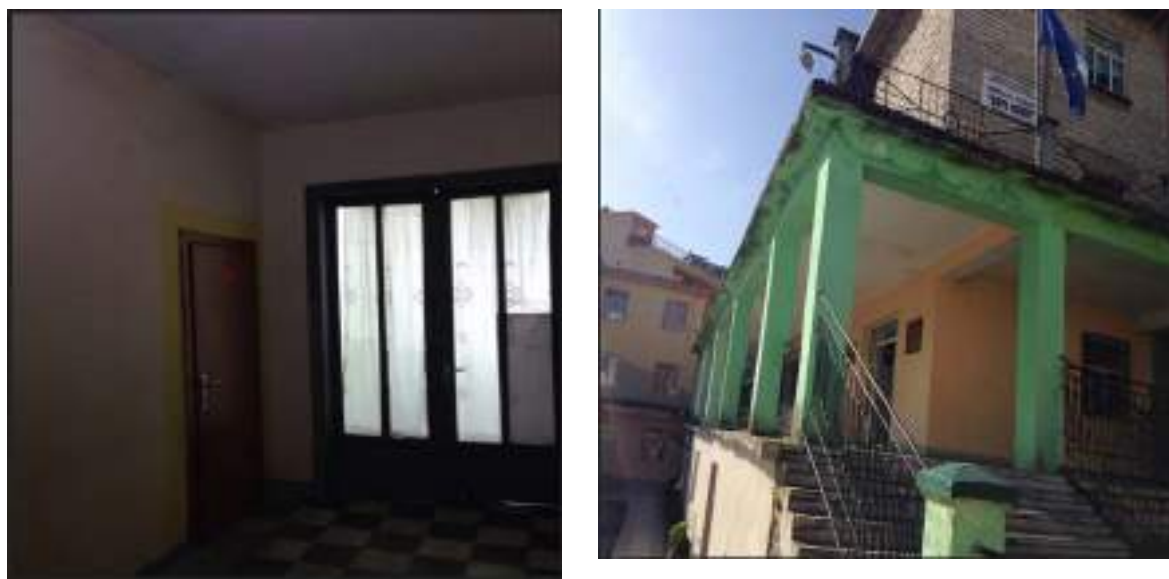
Figure 15-16: Pictures of the wall of outside doors
