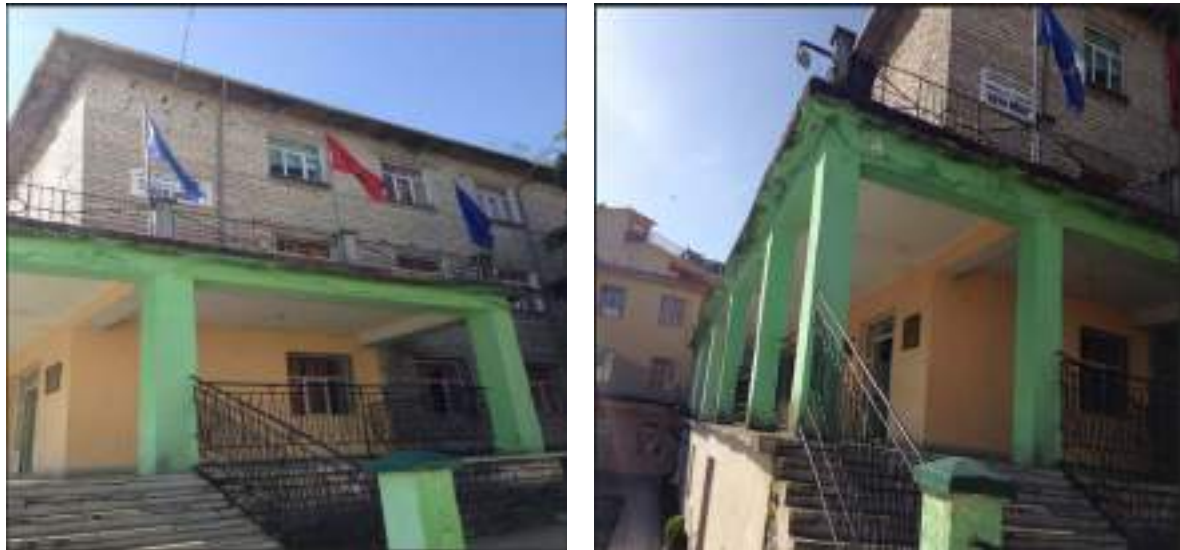
Figure 10-11 : Outside walls of the building
